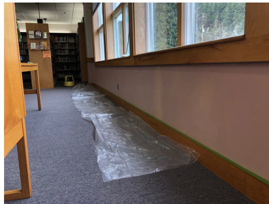
LIBRARY WALLS BEFORE PAINTING
